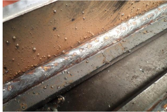
Fig-4 Spatters on weld
