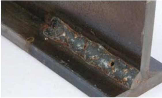
Fig-2 Porosity on weld
